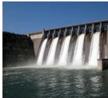
Shafts for water turbines
